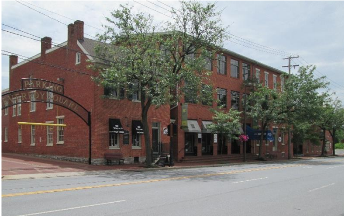
STREET VIEW OF BUILDING
